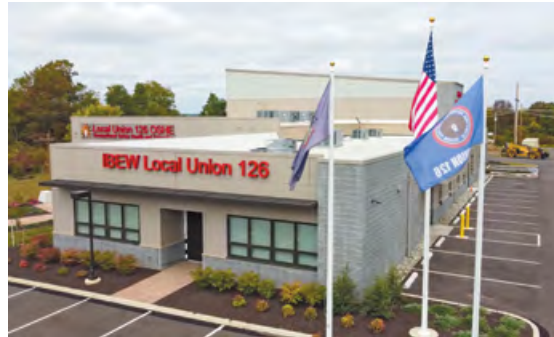
Local 126's newly renovated Collegeville union hall and training center.
